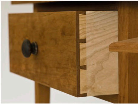
DETAIL OF THE LAPPED DOVETAIL
